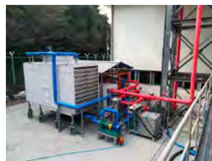
Heuksan (South Korea) - Heat recovery from thermoelectric power station (heavy oil gensets)
